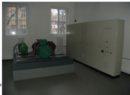
Fig.2. The wind generator system in the university laboratory.
